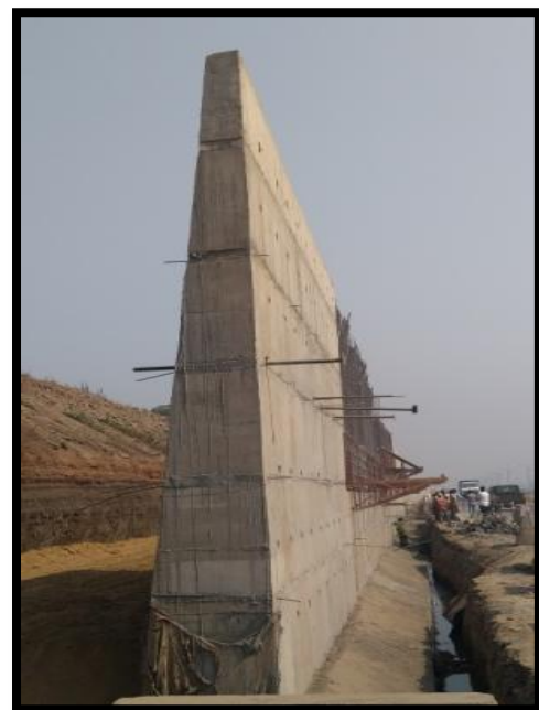
Fig. 9. Concreting Done up to Full Height for a Part of the Retaining Wall Length
