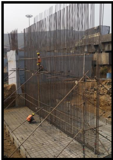
Fig. 11. A Complete Detailing of Reinforcing Steel
