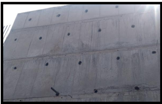
Fig. 12. A View of Outer Face (Non-Soil Face) Showing the Number of Weep Holes for an Effective Drainage
