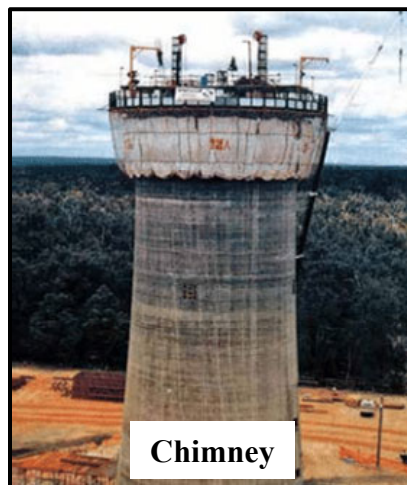
Fig. 3.13: Slip-form for a chimney under construction
