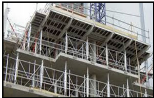
Fig. 3.8: Staging for slab
