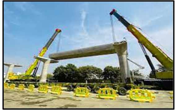
Fig. 3.31: Erection of full span by two cranes
