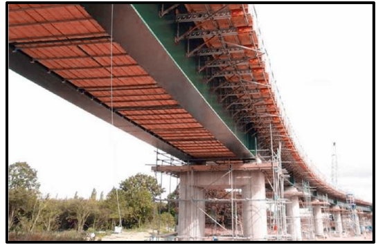
Fig. 3.29: Temporary formwork for the casting of deck slab
