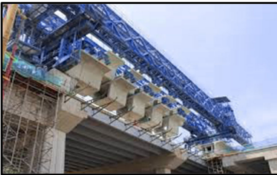
Fig. 3.33: Lifting of precast segments
