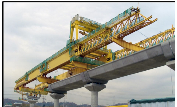
Fig. 3.34: Segmental span lowered onto the bearings
