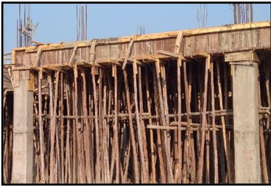
Fig. 3.10: Traditional / conventional formwork system
