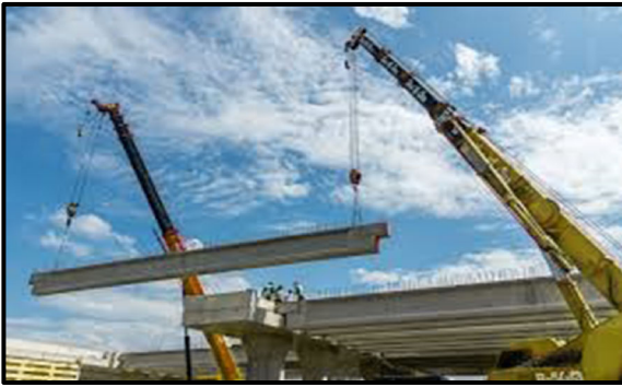
Fig. 3.28: Erection of girders with crane
