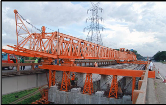
Fig. 3.30: Launching girder for girder erection
