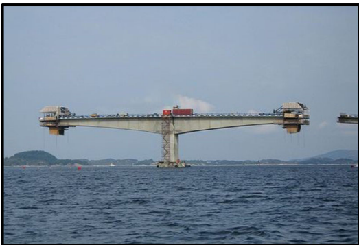
Fig. 3.36: Balanced cantilever construction using precast segments
