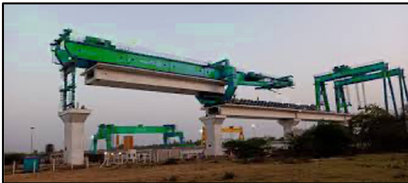
Fig. 3.32: Full span launching of girder
