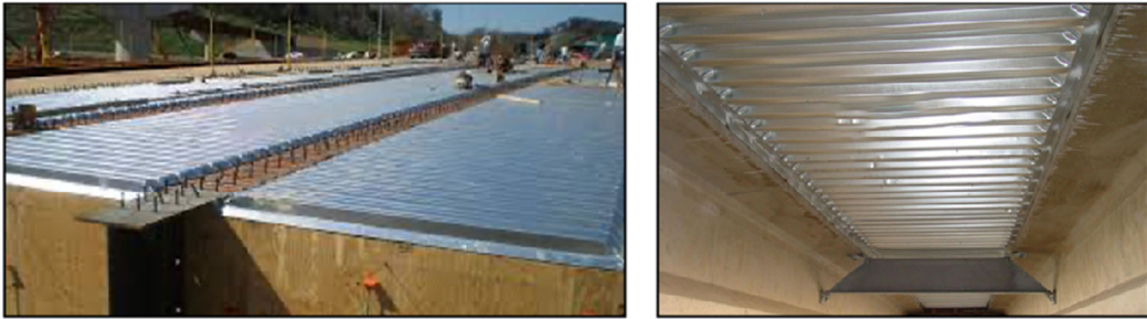
Fig. 3.9: Rolladeck left-in-place formwork
