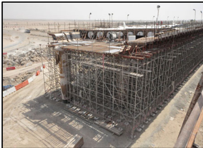
Fig. 3.27: In-situ construction using ground-supported formwork system
