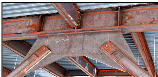
Fig. 3.24: Welded joint
