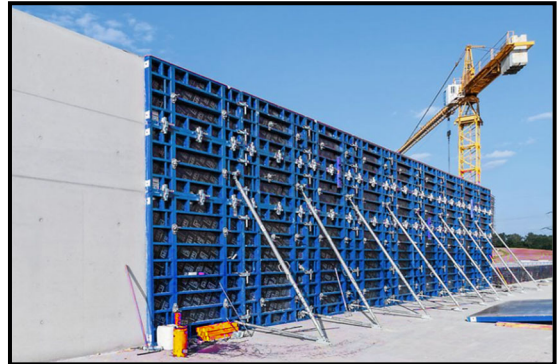
Fig. 3.11: Engineered formwork system
