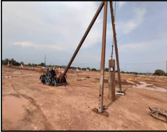
Fig. 3.3: Bailer and chisel with tripod and winch
