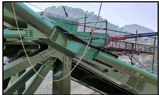
Fig. 3.23: A bolted joint in a bridge
