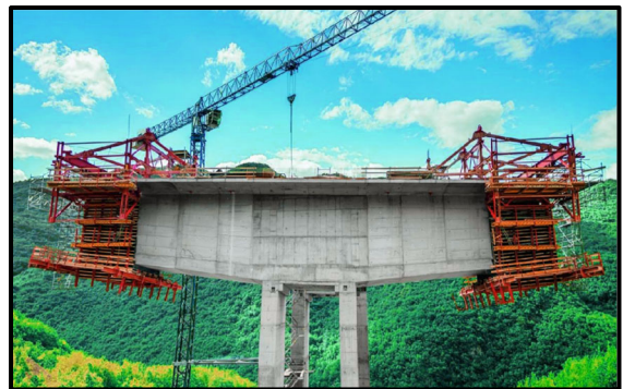
Fig. 3.37: Balanced cantilever construction using cast in-situ segments
