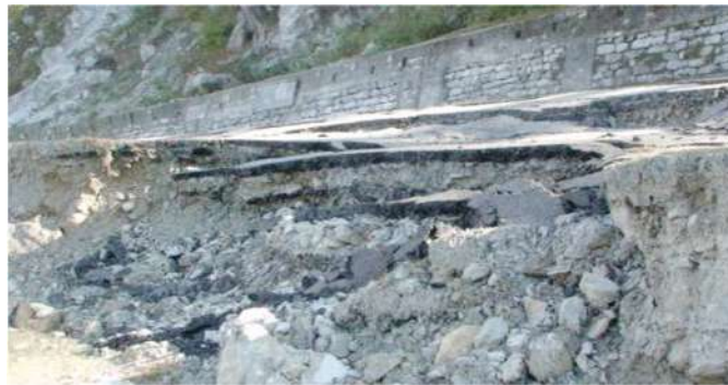
Fig. 2.38: Example of lateral spreading
