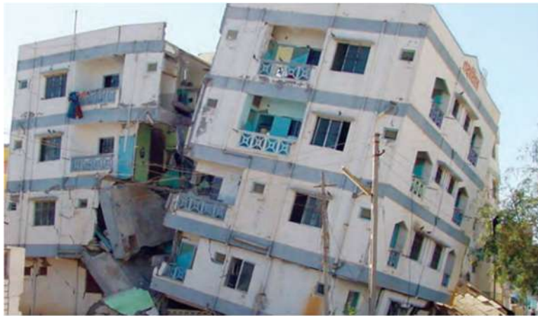
Fig.2.1: Building damaged due to Gujarat 2001 earthquake
