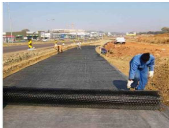
Fig. 2.9: Use of Geotextile in road construction
