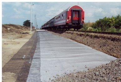
Fig. 2.10: Use of geotextile in railways
