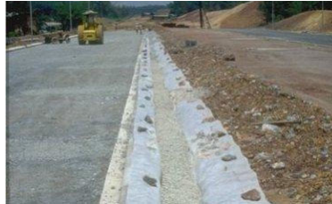
Fig. 2.11: Use of Geotextile in drain construction
