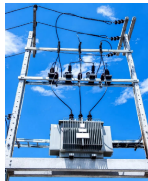
(b) Pole-mounted Distribution Transformer
