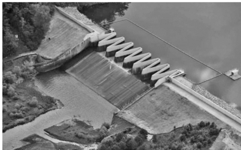
Figure 5.10 Labyrinth weir (after Crookston and Tullis, 2013)
