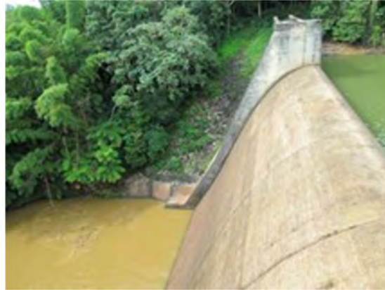
Figure 3.27: Ogee spillway (Cidra Dam)
