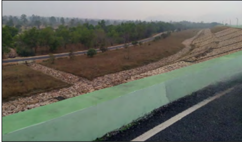
Figure 3.7 Downstream pitching, Rock toe, and toe drain in right dyke of Hirakud Reservoir
