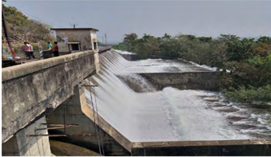
Figure 3.43: Stilling basin after flowing over the weir upstream of Chiplima power house, Odisha
