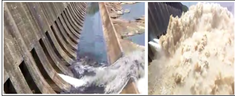
Figure 3.38: Trajectory Bucket type / Sky Jump energy dissipator
