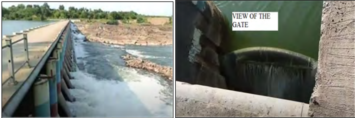
Figure 5.6 Standard K.T Weir Gates
