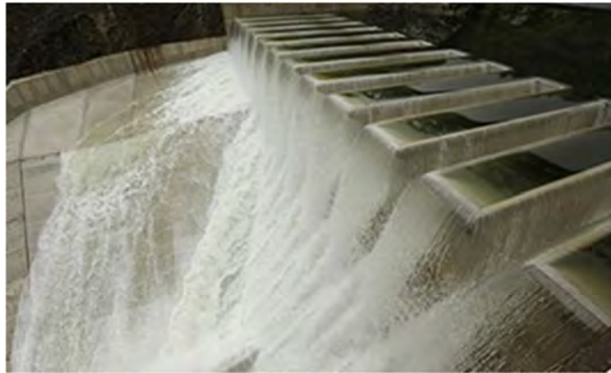
Figure 5.11 View of Piano-Key Weir
