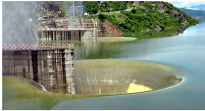
Figure 3.31: Shaft Spillway of Tehri Dam on River Ganga
