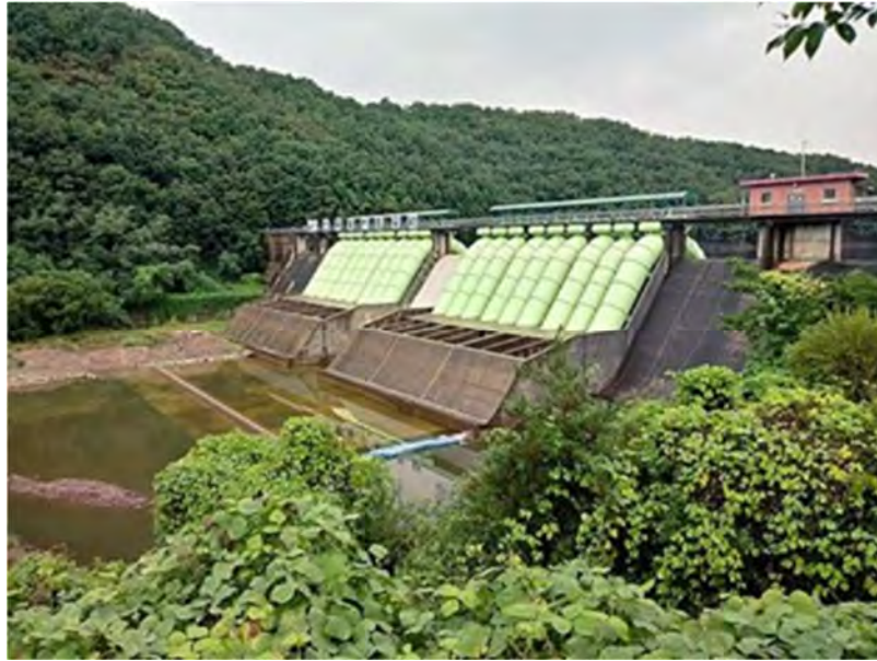
Figure 3.34: Siphon spillway (Chopyeong Dam)
