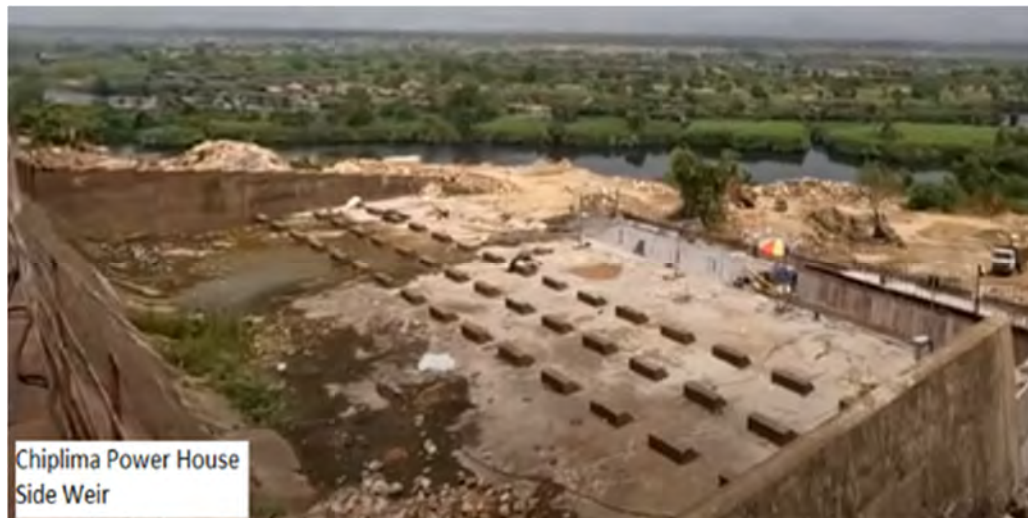
Figure 3.42: Stilling basin (View during Maintenance work) at downstream of the weir at Chiplima power house
