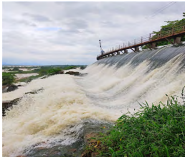
Figure 3.29: Side Channel spillway
