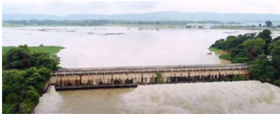
Figure 3.33: Siphon Spillway releasing excess water from the Power channel
