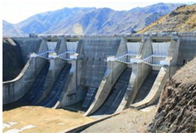
Figure 3.28: Chute spillway (Benmore Earth Dam)
