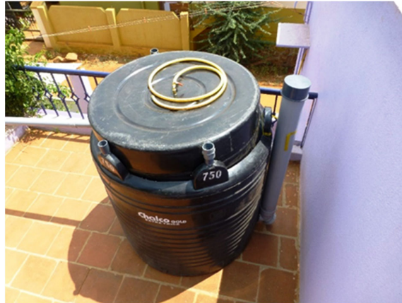
Fig.3.59 Fixing the feed pipe to the digester
