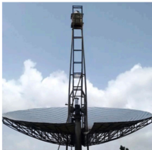
Fig.3.47 Receiver support structure
