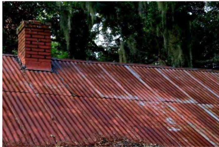
Fig. 5.4: UNIFORM CORROSION OF METAL ROOF
